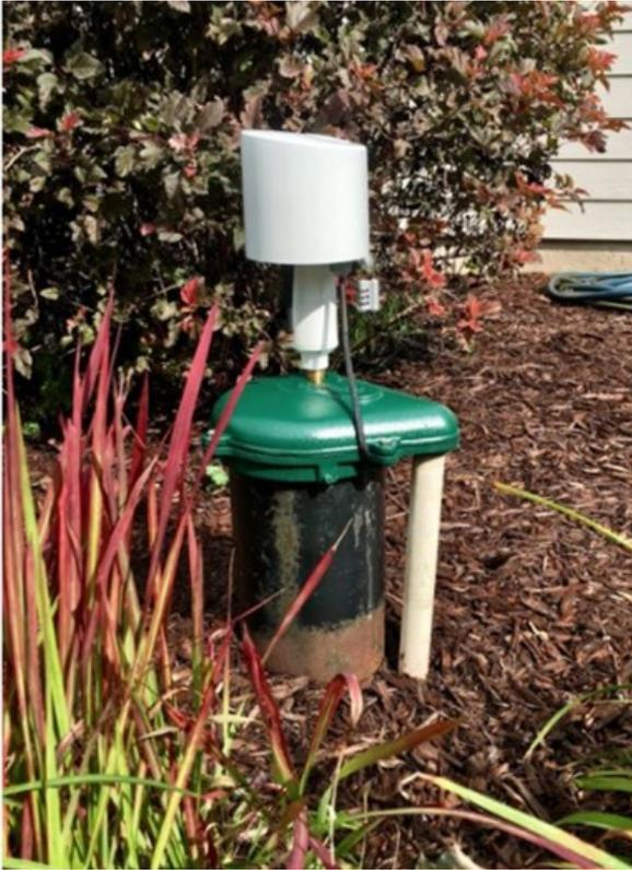
*Typical installation of the homeowner well water-level monitoring system.*
